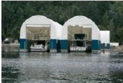
Fire retardant Spider Weave fabric is standard on all installations to make use of natural light and can be tailored to individual requirements to allow for insulation. Custom fabrics are available for specialty use applications or local considerations.
